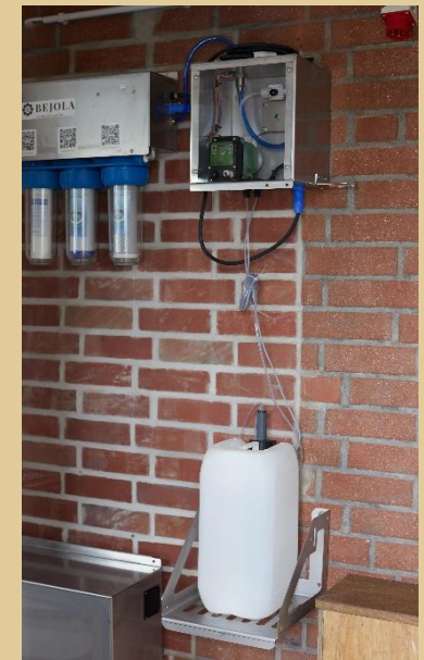
Bejola Spraying Systems with one dosing unit. Up to 3 dosing units can be installed.
